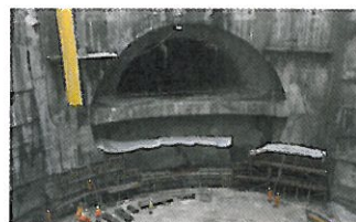
Construction of Abu Dhabi's huge new sewer system
