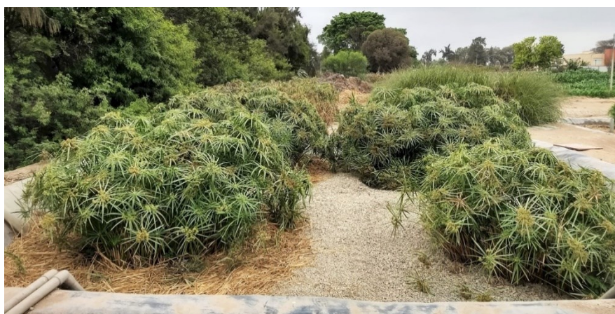
Figure 2: Pilot in Lima/Peru plant with 1 st stage for raw wastewater treatment, the left line is covered with a layer of sawdust and chopped plants, and in the background 2 nd stage, two parallel operated vertical flow filter
